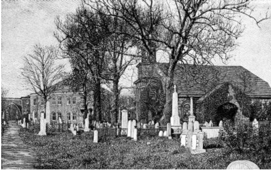
Old Swedish Church at Wilmington, Delaware.
